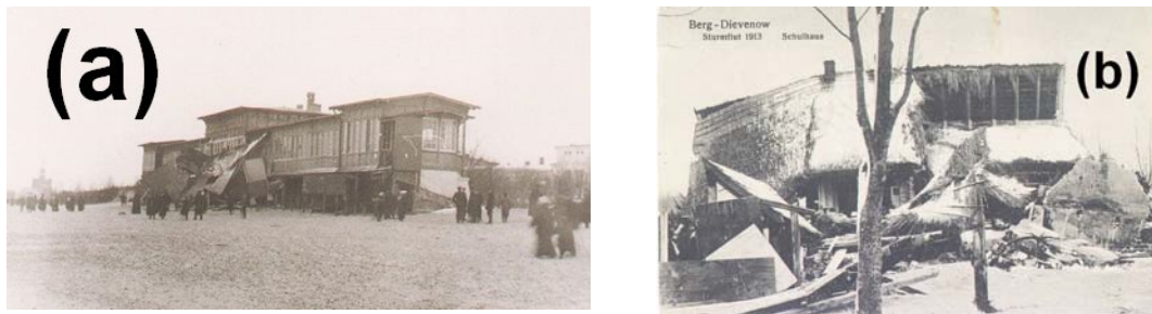
Figure 13. Postcards showing damages in in Dziwnów, Poland, caused by the storm surge on 30 December 1913.
